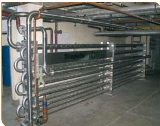
Waste water heat recovery saves 15%.
